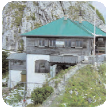
Electricity for mountain cabins
